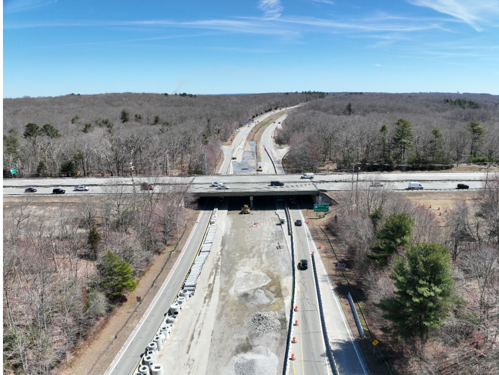
Corridor - Tower Hill Rd.
